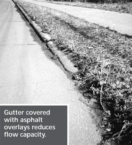
Gutter covered with asphalt overlays reduces flow capacity.
