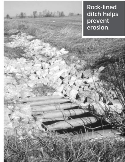
Rock-lined ditch helps prevent erosion.
