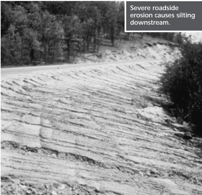
Severe roadside erosion causes silting downstream.
