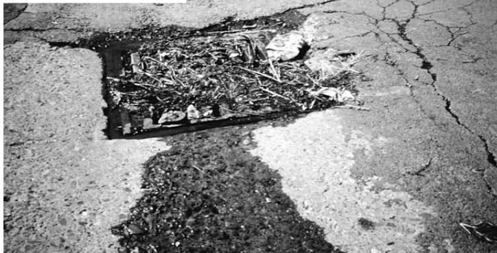
Pavement settlement causes ponding in this poor parking lot inlet.
