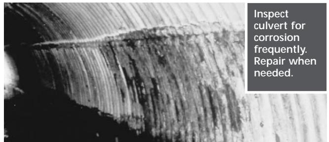
Inspect culvert for corrosion frequently. Repair when needed.
