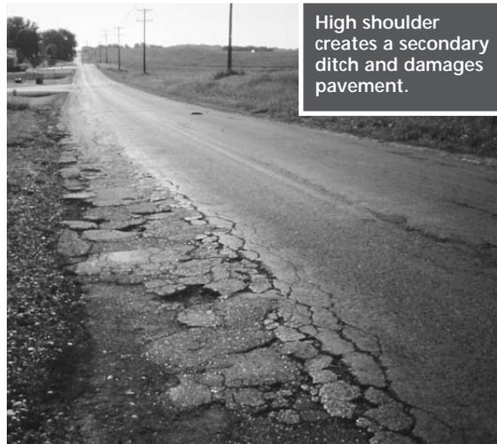
High shoulder creates a secondary ditch and damages pavement.
