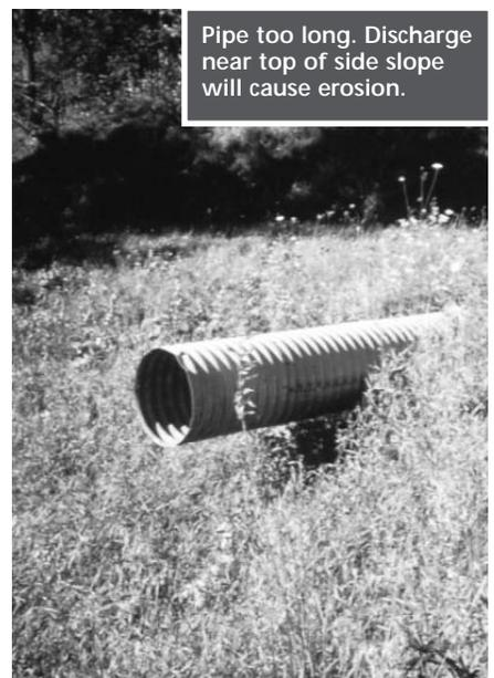
Pipe too long. Discharge near top of side slope will cause erosion.
