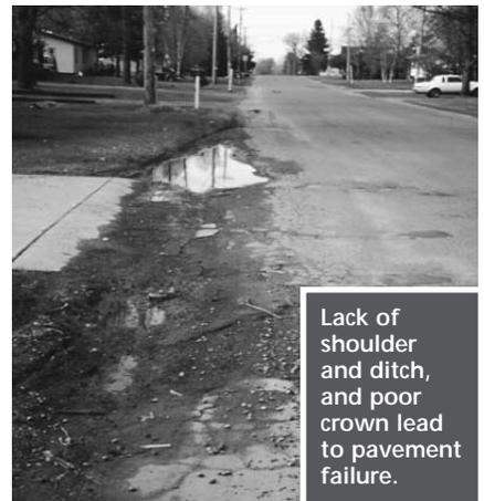
Lack of shoulder and ditch, and poor crown lead to pavement failure.
