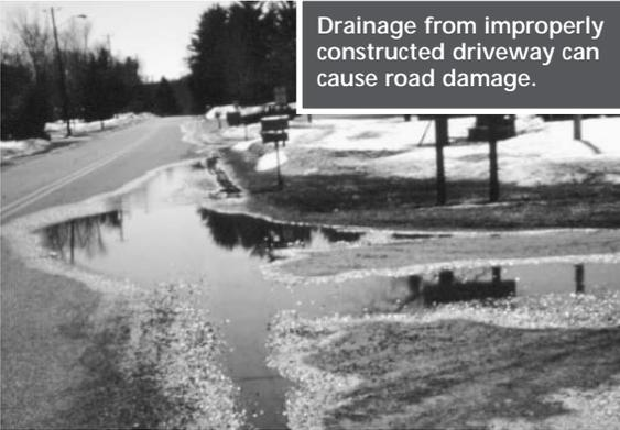
Drainage from improperly constructed driveway can cause road damage.
