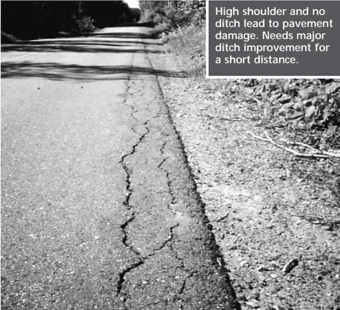
High shoulder and no ditch lead to pavement damage. Needs major ditch improvement for a short distance.
