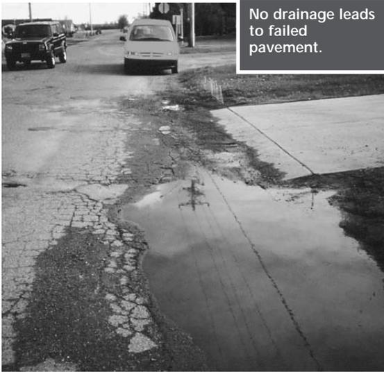
No drainage leads to failed pavement.
