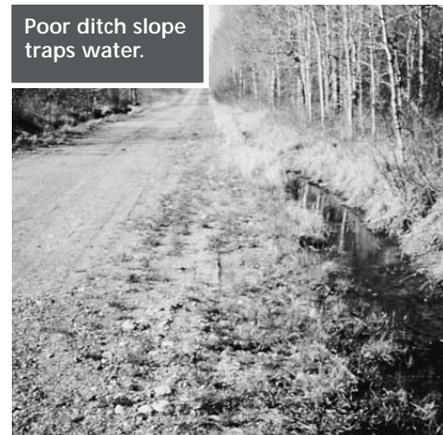
Poor ditch slope traps water.
