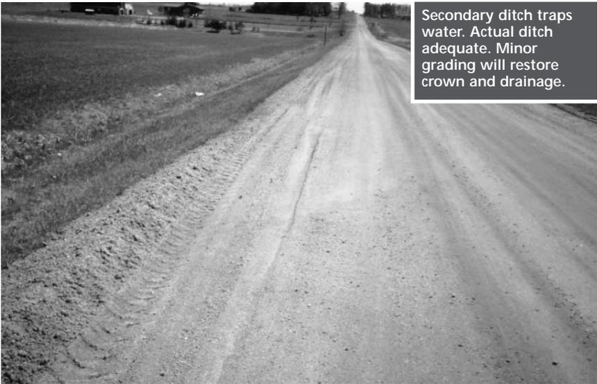
Secondary ditch traps water. Actual ditch adequate. Minor grading will restore crown and drainage.
