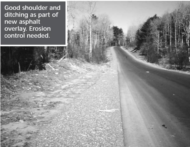
Adequate ditch and good erosion control.
