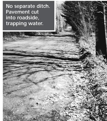
No separate ditch. Pavement cut into roadside, trapping water.
