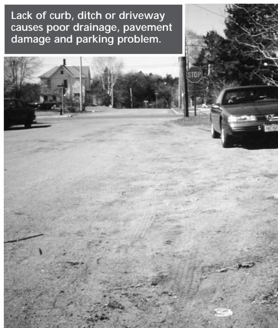
Lack of curb, ditch or driveway causes poor drainage, pavement damage and parking problem.
