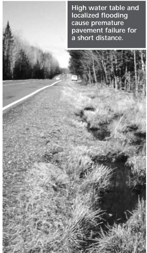
High water table and localized flooding cause premature pavement failure for a short distance.
