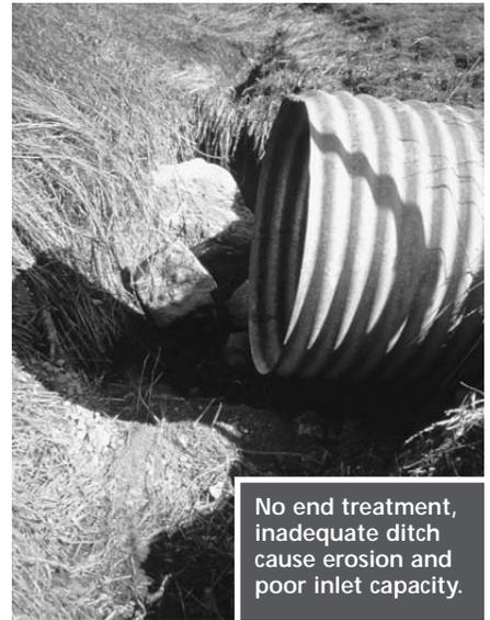
No end treatment, inadequate ditch cause erosion and poor inlet capacity.
