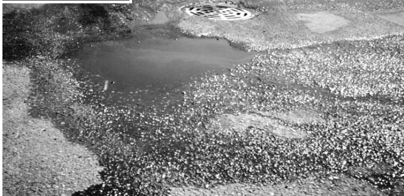
Clogged inlet causes flooding.
