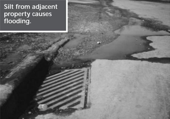
Silt from adjacent property causes flooding.
