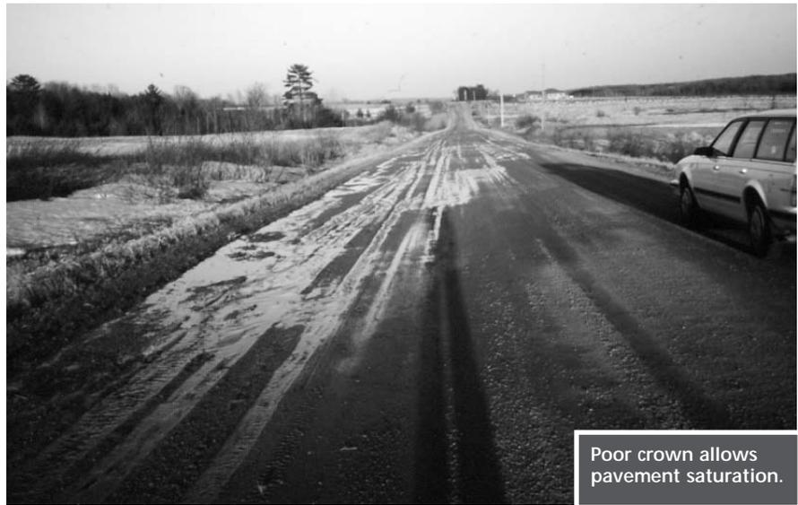
Poor crown allows pavement saturation.
