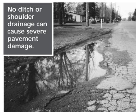
No ditch or shoulder drainage can cause severe pavement damage.
