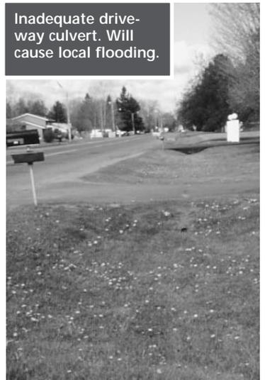
Inadequate driveway culvert. Will cause local flooding.
