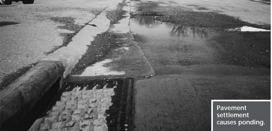
Pavement settlement causes ponding.
