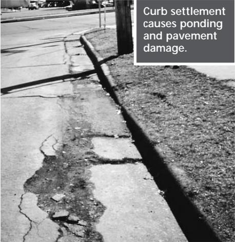
Curb settlement causes ponding and pavement damage.
