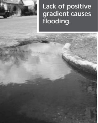
Lack of positive gradient causes flooding.
