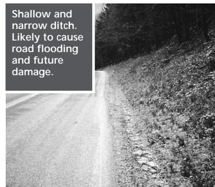
Shallow and narrow ditch. Likely to cause road flooding and future damage.
