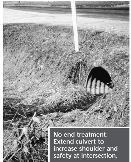
No end treatment. Extend culvert to increase shoulder and safety at intersection.
