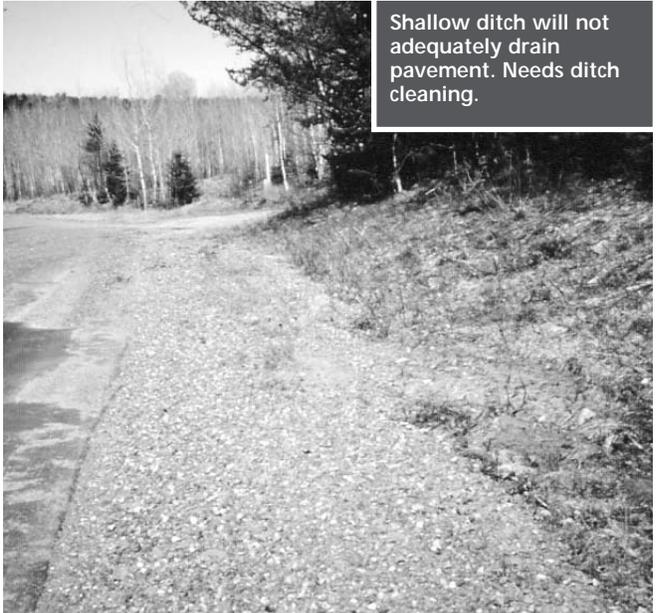
Shallow ditch will not adequately drain pavement. Needs ditch cleaning.
