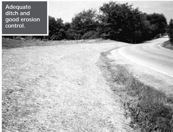
Good rural ditch and driveway culvert. Culvert end needs cleaning.
