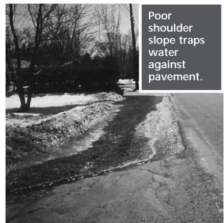
Poor shoulder slope traps water against pavement.
